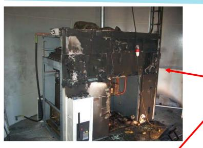
OVERVOLTAGE: short circuit in one electrical panel. Source:
